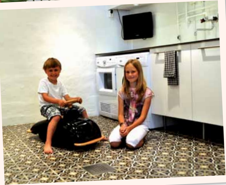
Erik & Ebba in their newly renovated laundry room. The family is now happy to spend time in the laundry room. Warm floors and a TV make ironing and folding washing more enjoyable.
